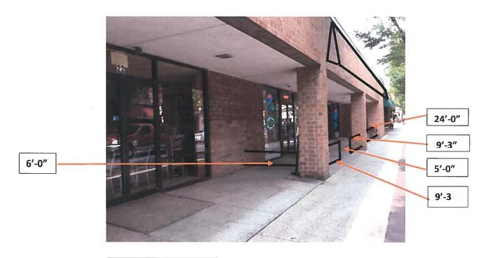
Height to underside of recess is 9'-4" +/-
