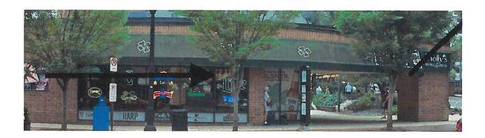
1.Replace existing awning with new fabric on existing galvanized frame at 8 4th St. Awning to have open ends. Black Sunbrella fabric with Molly's logo centered on each section of awning. Background will be black. Length 49'-3"
