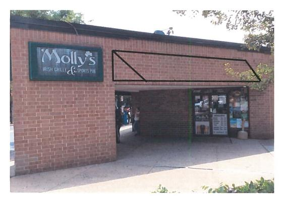
1.Install new awning above opening at 8 4<sup>th</sup> Street rear. Awning to be the same configuration as 4<sup>th</sup> Street elevation (There was an awning at this elevation at some point as fasteners are still on building). Length will be 27'-4" Awning fabric to match 4<sup>th</sup> street awning.
